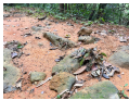
The gully on this section of road was eventually repaired with a stone road made of large rocks.
