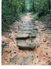
The gully on this section of road was eventually repaired with a stone road made of large rocks.
