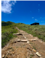
In 2024, some gentle stone steps were added to the same section of hiking trail, making it safer for hikers.
